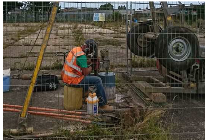
Figure 11: Photograph of ground investigations on site
