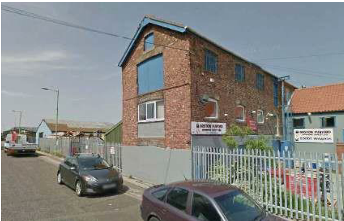
Plate 9-12 – Warehouse at 41 Commercial Road
