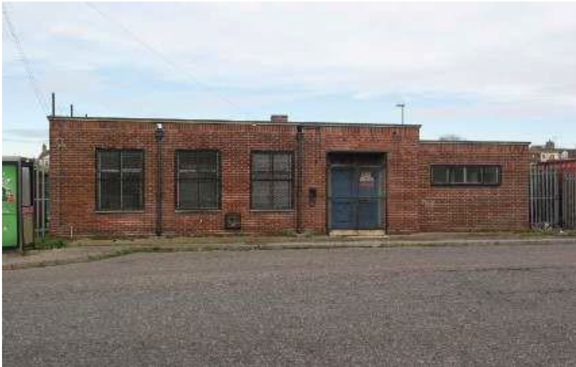
Plate 9-14 – Freight Yard Building, Commercial Road
