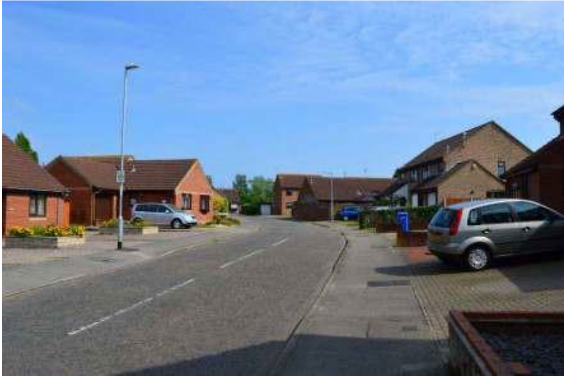
Plate 10-15 – Mixed housing along Planters Grove in Coleville in the south of the LCA LCA 8 Oulton Broad
