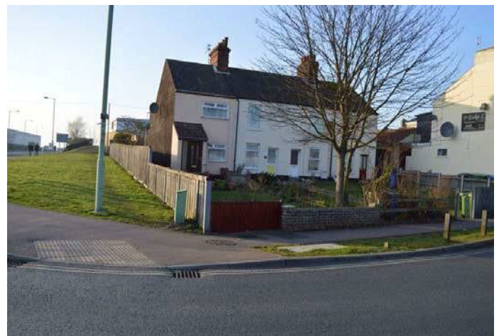
Figure 13: Photograph residential properties adjacent to the site
