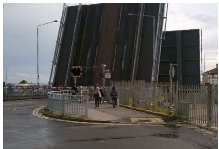
Figure 3: Photograph showing existing bascule bridge while open
