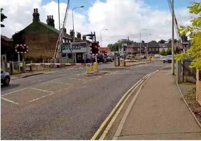
Figure 19: Photograph showing level crossing barriers and lighting
