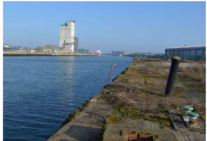
Figure 14: Photograph of existing conditions on proposed crossing location
